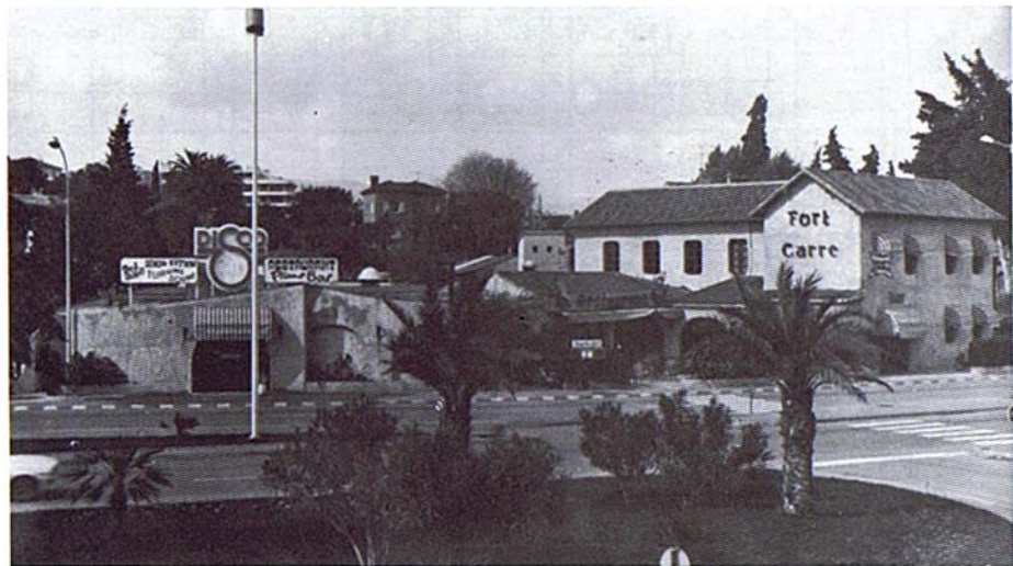
SOURCE DIRECTION FORT CARRE
